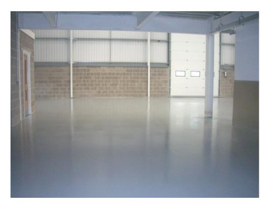
EPOXY PRODUCTS EPOXY COATING SB is an extremely tough, chemical resistant, inexpensive two-pack, solvent based epoxy resin coating for concrete and wood flooring.
